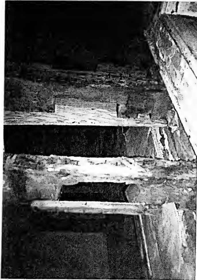
Figure 14: Joists along the first floor ceiling of the Pawling house
